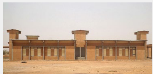
Solar chimneys, Luxembourg Cooperation in Niger, 2016 Source: LuxDev (2016), bioclimatic construction in Niger
